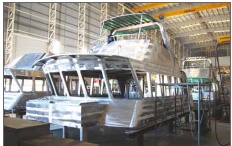
▲ The 21.2m inshore patrol craft under construction in Henderson, Western Australia.
